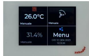
The ventilation unit takes the minimum fan speed as default. Via the relays it contains, Multi Control activates the second and third fan speeds when requested by the user or when necessary to meet post-treatment needs.
