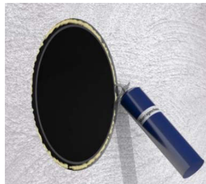
Fig. 5 Sealing the wall mounting pipe
