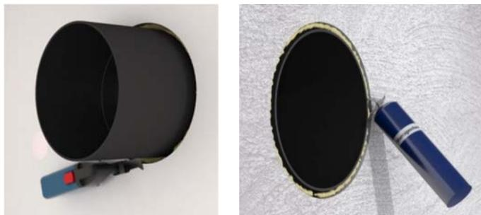
Position the bottom cover of the exterior wall panel centrally on the PVC wall mounting pipe, maintaining a distance of  $x = 33 \text{ mm}$ , and align it horizontally with the façade. Transfer the drill holes and prepare a suitable fastening technique for the four fixing points (shown as long holes) as set out in the façade design.
